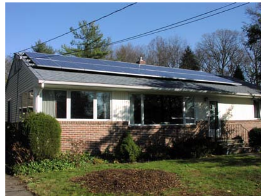
Figure 1: The PV array of 2 branches of 12 Sharp ND-216 UC1 PV modules,
